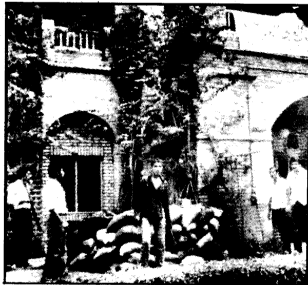
Above: Workers in Khoramsha in the province of Khuzestan defend a building against the attacks of the Islamic militias.
